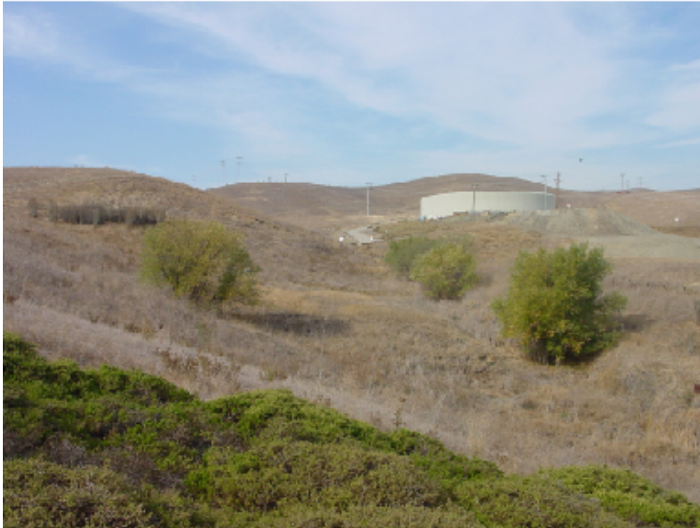
Viewpoint 3: Reservoir Site from property line at 109 Shireoaks Place looking northwest.
