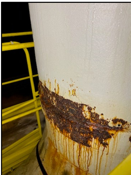
Force Main Before Recoating
